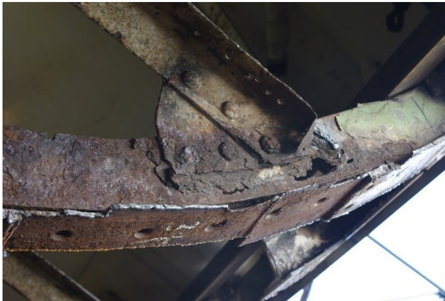
Frame corrosion Jeff Malley
