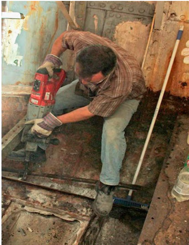
Using a jack hammer to remove concrete Jeff Malley
